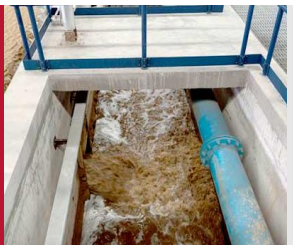
Water treatment plant, Tianjin, China
