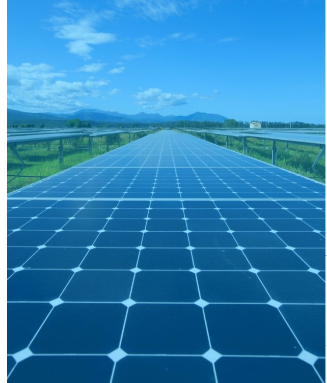
Photovoltaic power plant – Porette de Néron, France
