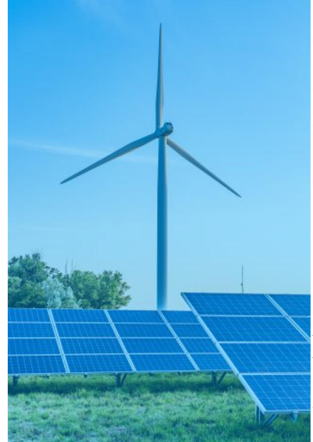
Photovoltaic power plant – Bollène, France
