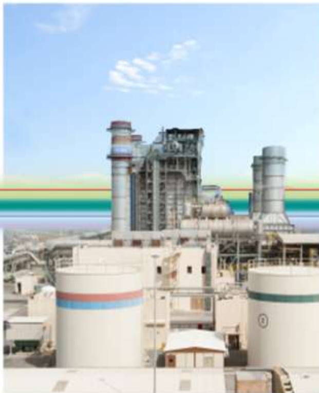
Power & desalination plant, Barka 2, Oman
