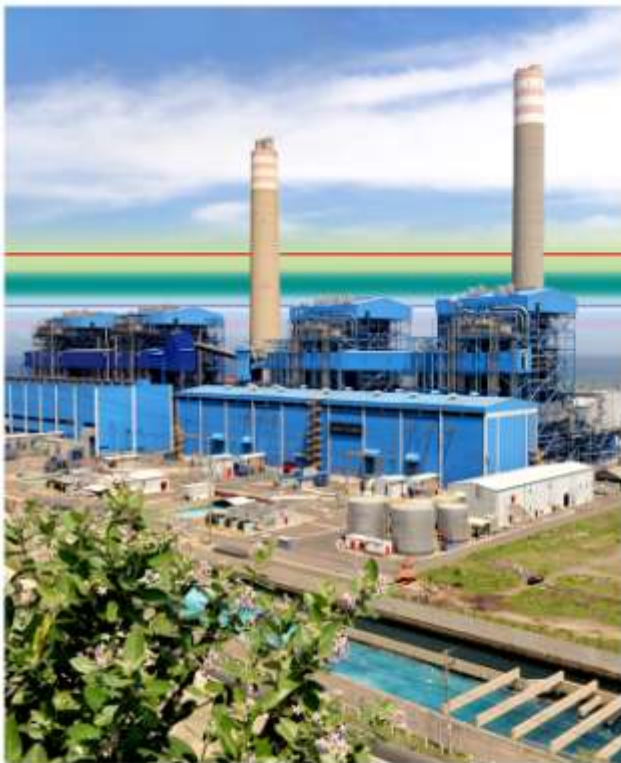
Paiton coal power plant, Indonesia
